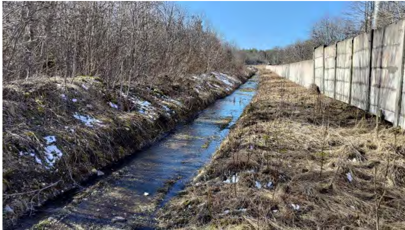
Figure 2.3. Drainage ditch at the PAL site.
