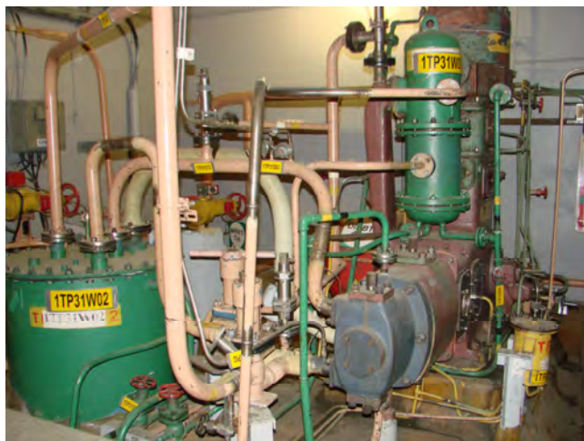
Gaseous circuit. Helium compressor.
