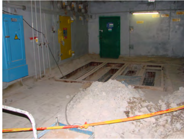
Installation of the transportation aperture
