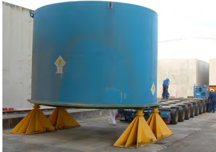
Reactor vessel head (removal, disposal and injection)
